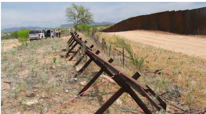
Vehicle barrier on Buenos Aires National Wildlife Refuge. Pronghorn antelope and other threatened species are able to cross the vehicle barrier but not the solid pedestrian fence to the right.
